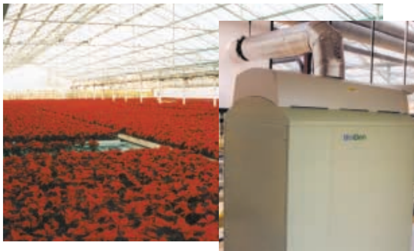
W.J. Findon & Son greenhouse located in Stratford-upon-Avon, UK, takes advantage of the very clean exhaust and CO 2 .
