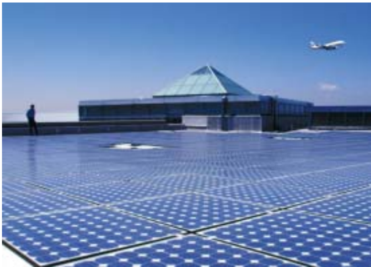
Installation of PowerLight photovoltaic panels atop a Los Angeles corporate building.
